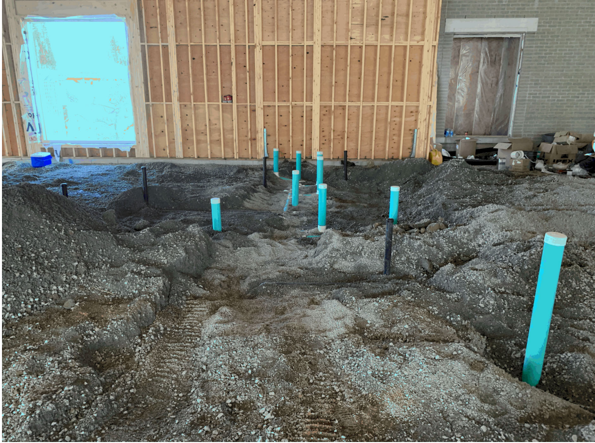
Figure 2: Daycare Addition Construction – Underground Plumbing Installation
