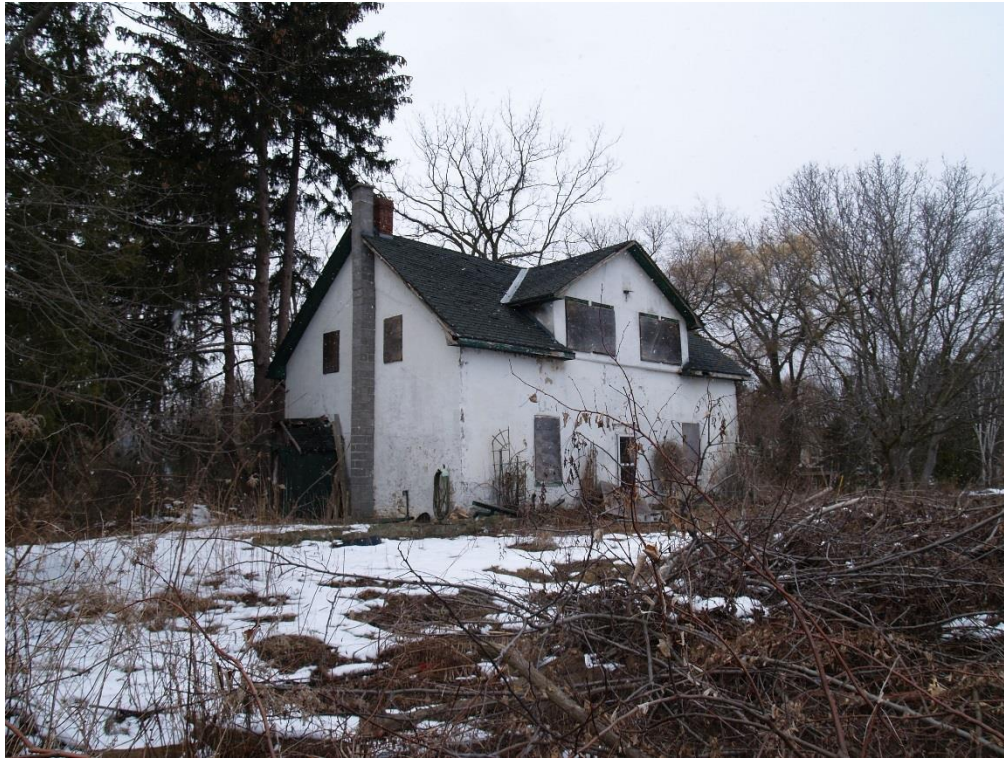
Figure 3: View facing northwest of Secord-Paxton House and its surrounding thick vegetation (2018).
