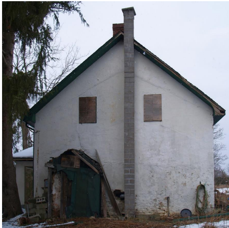
Figure 5: South end wall (2018, photographed with pole-mounted camera and rectified).
