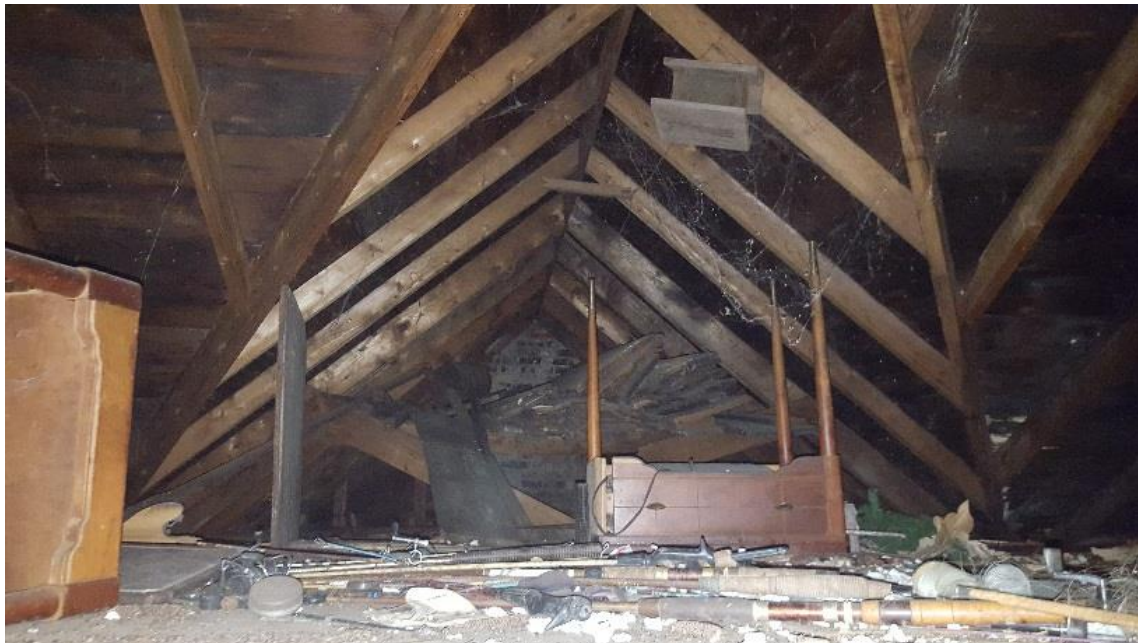
Figure 13: Attic space with exposed dimensional lumber common rafters and sheathing (2017).
