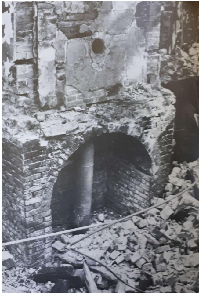
Figure 15: Large chimney base with relieving arch in Liston House, Delaware, circa 1740 (Herman 1987:90).
