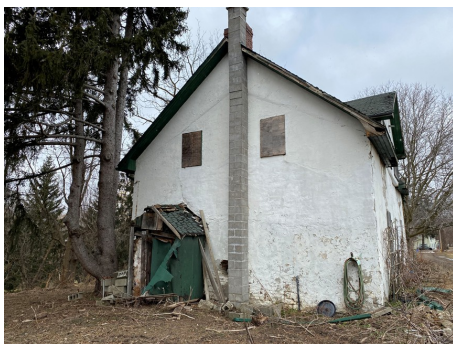
The new roof line
