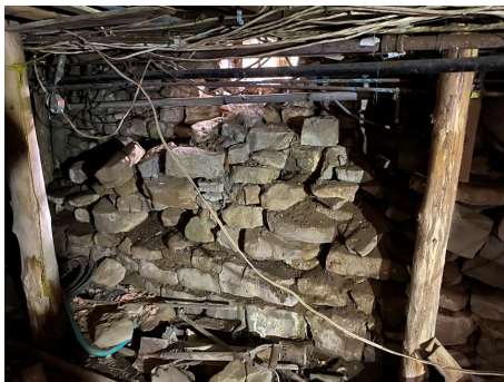
The stone wall without joint mortar
