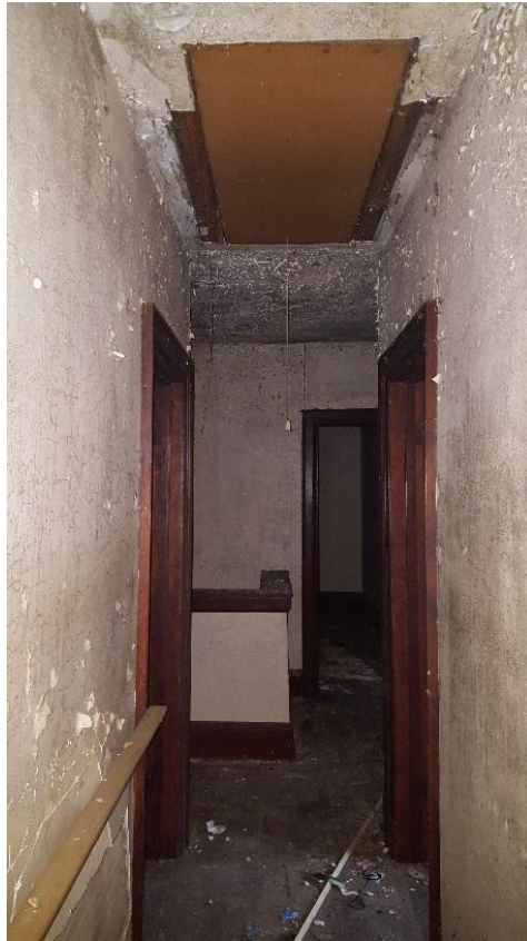
Figure 11: Second level hallway, facing south toward the staircase (2017).
