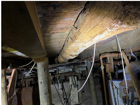
Old and new floor joist/post
