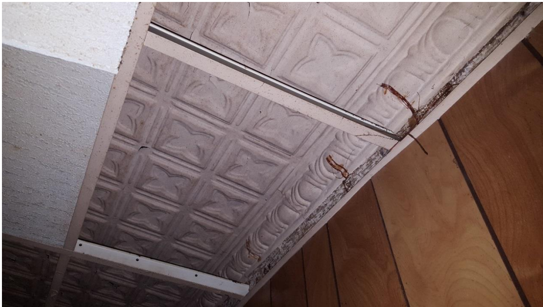
Figure 9: Pressed metal ceiling in the southwest room (2017).
