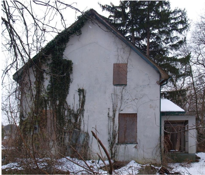
Figure 7: North end wall (2018, photographed with pole-mounted camera and rectified).
