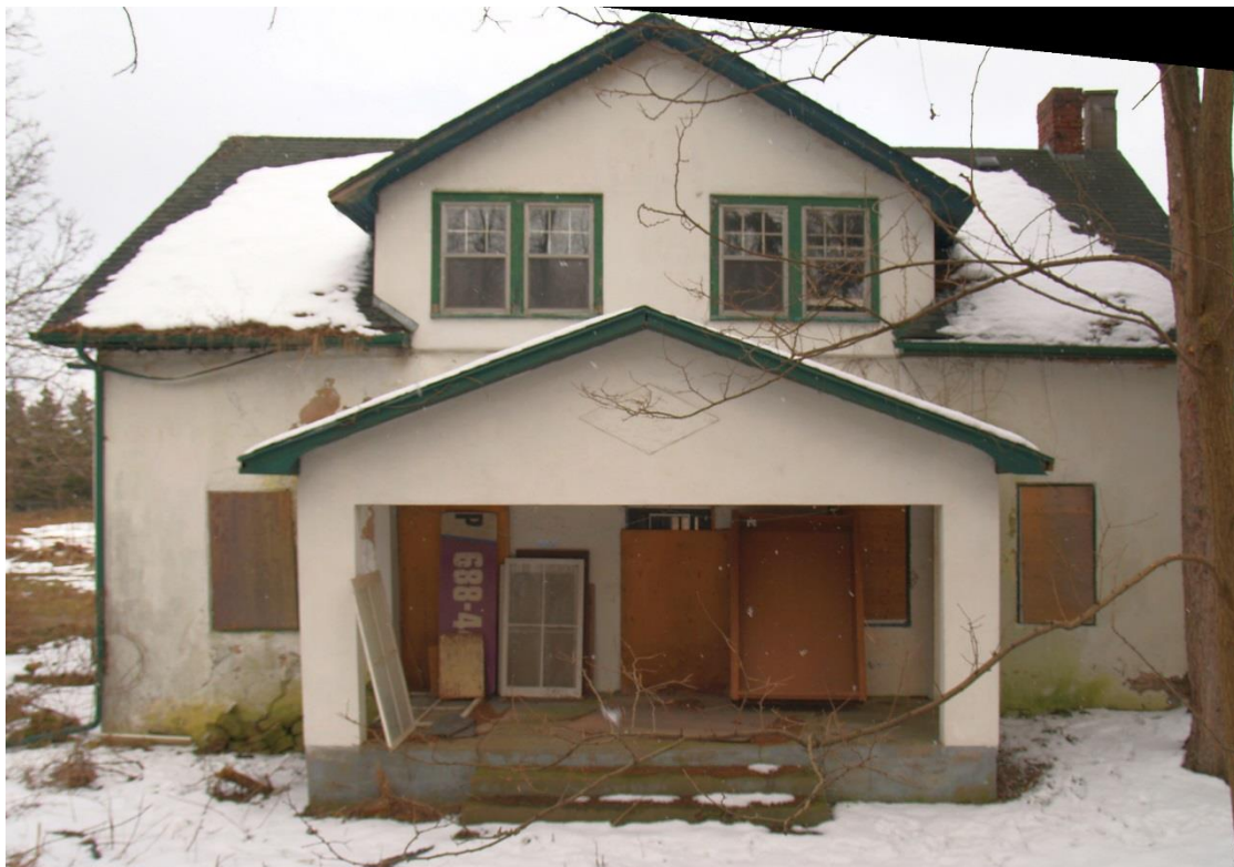
Figure 6: East façade (2018, photographed with pole-mounted camera and rectified).
