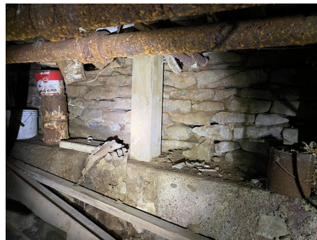
Benching at the bottom of the wall
