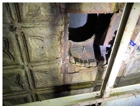
Exposed floor structure
