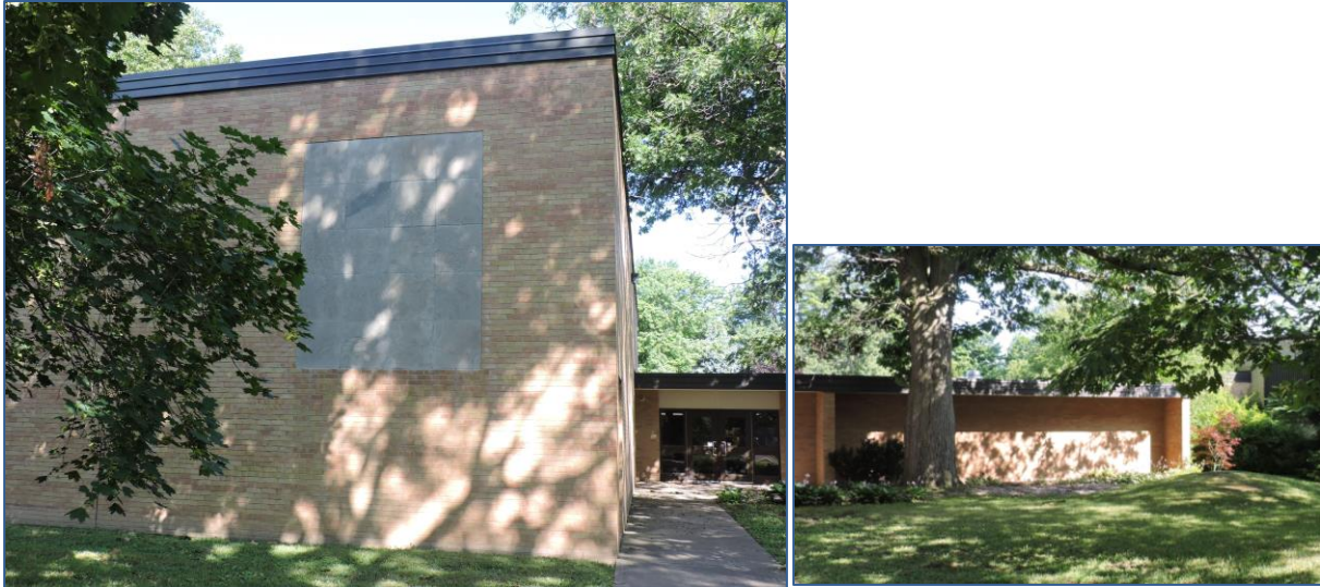
Figure 32: Gymnasium additions and the one storey link (AB, 2018).
