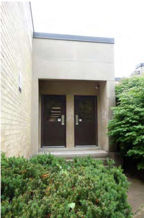
1947 original school – doors are not original
