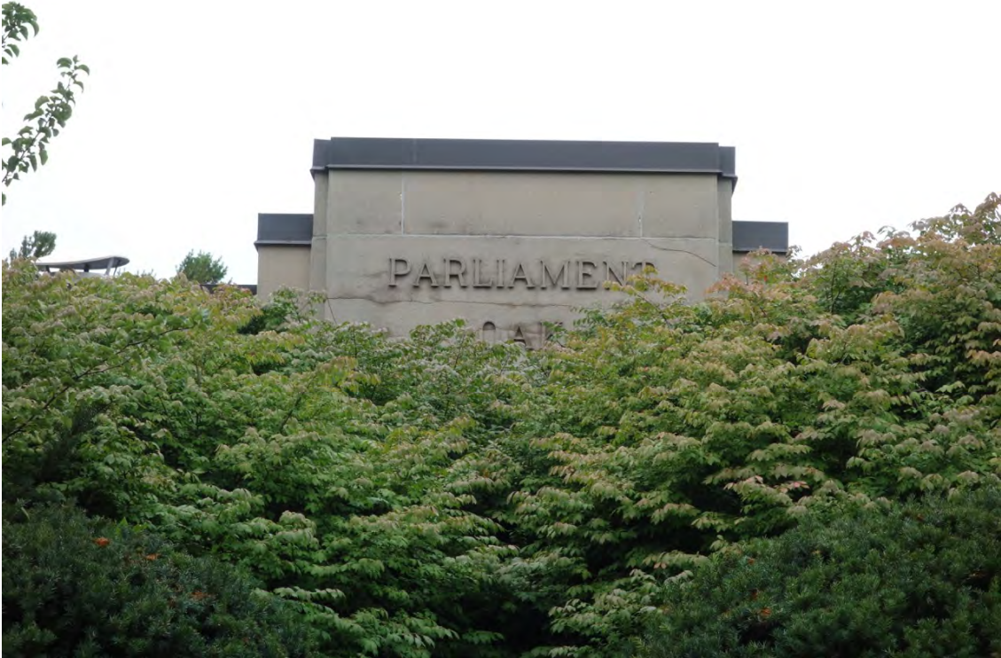
Carved stone lettering on the parapet, c. 1947
