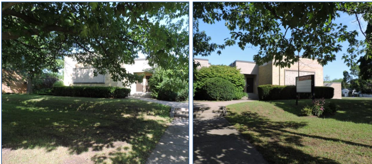
Figure 29: Front of building (AB, 2018).
