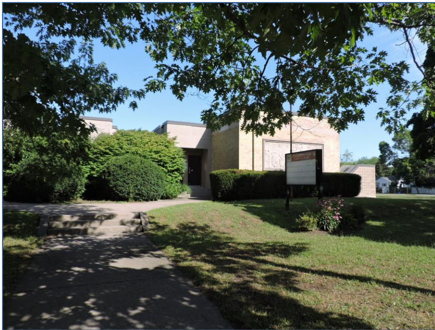
Figure 5: Part of the front façade (AB, 2018).
