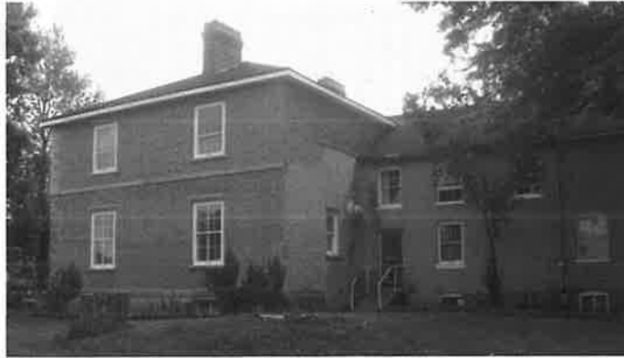
Locust Grove, roadside view today, with original brick exposed. (Courtesy: Author's Collection)
