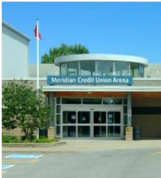
Figure 14: Entry to MCU Arena
