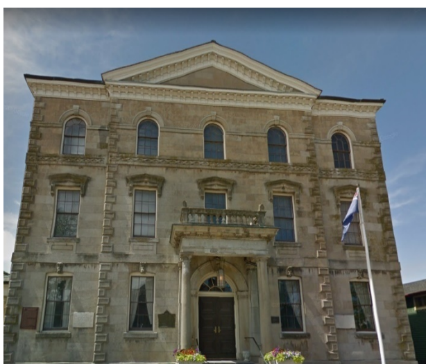
Figure 10: NOTL Historic Court House
