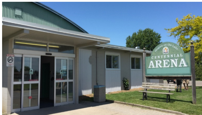
Figure 13: Entry to Centennial Arena
